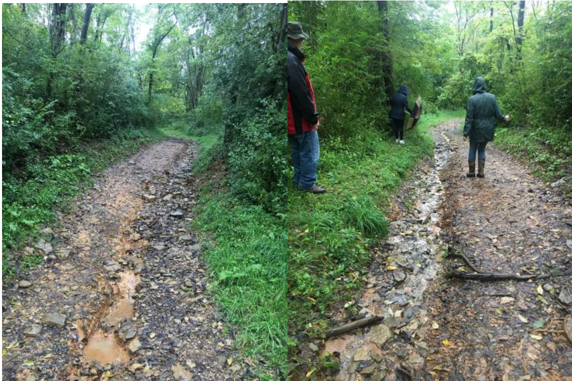
Figure 2.2. Major erosion at the start of the trail. On the left is looking up the trail. On the right is the same location in the trail but looking down the slope.
