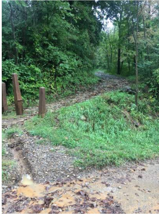
Figure 2.1. Erosion and gully forming at the trailhead
